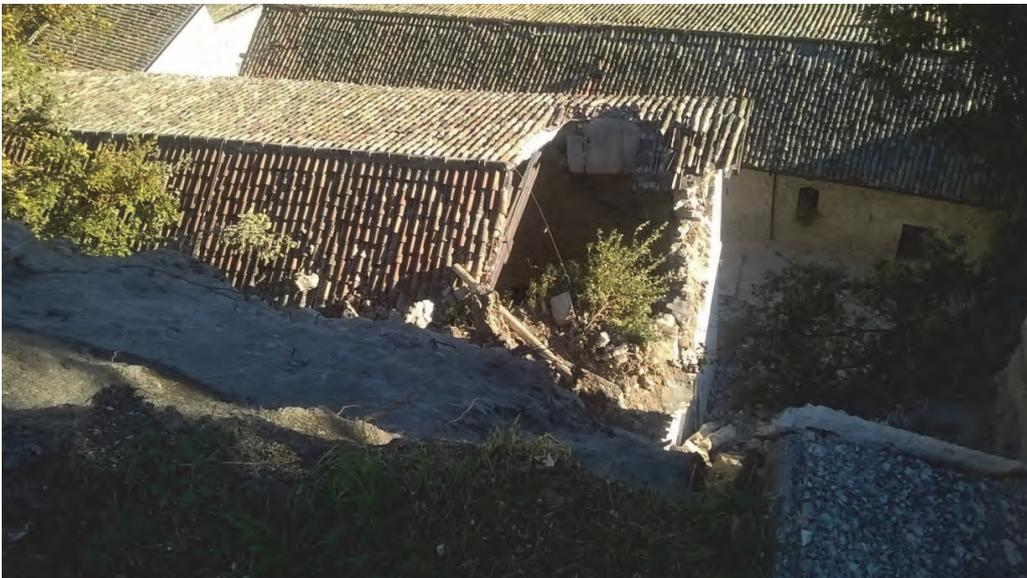
Seminar structure damaged by the collapse of the funeral shrines and part of the travertine plate.
