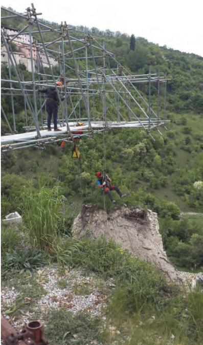
Descent from above of the operators in charge of removing the travertine pinnacle.
